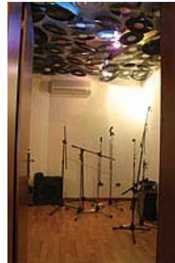
The first thing you notice in the first live room is that the only permanent acoustic treatment is provided by vinyl LPs screwed to the ceiling through short lengths of plumbing pipe cut at an angle, so that the LPs are not parallel to the ceiling (see photo, above centre). A tastefully covered mattress provides a piece of movable treatment, as does a thick rug. Future plans include providing fixing points for either heavy curtains or duvets, so that the room can be damped down when necessary.
